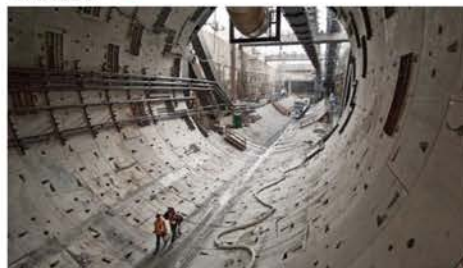
This tunnel is 57.5' in diameter, a little bigger than the two 40' tunnels planned to deliver the Sacramento River, but you get the idea.
