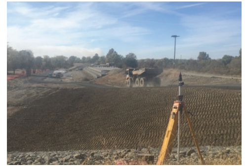
Heavy equipment at work grading restored habitat for salmon
